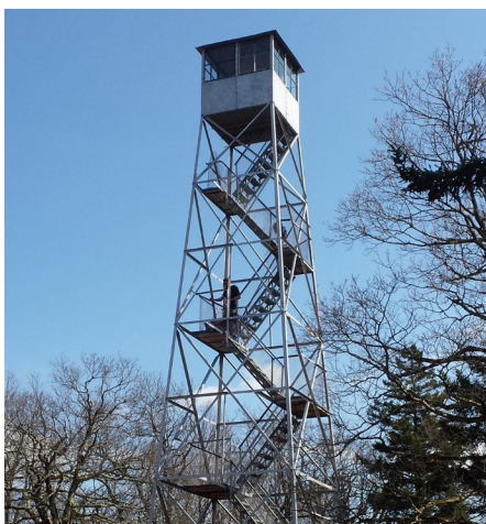
Photo contributed by the Basket Historical Society The Red Hill fire tower in Denning, NY, near Claryville. Once, spotters watched for forest fires from towers like this. (During wartime, spotters watched for enemy planes, too.) The Red Hill tower is 60 feet tall and was built in 1921. As with all the Catskills fire towers, it was used less over time; fire-spotting from the air was more efficient. The tower finally closed in 1990.
